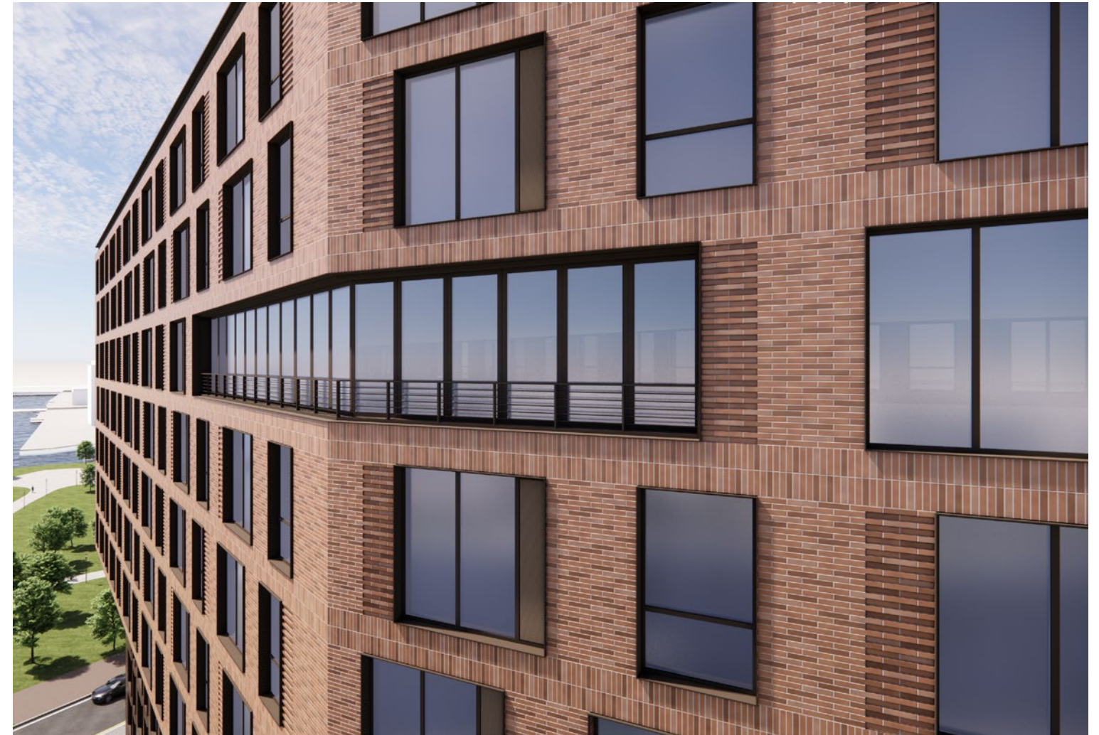
VIEW OF FACADE AT AMENITY SPACE
