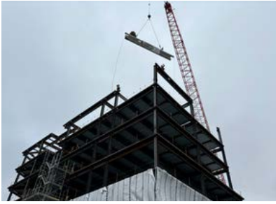
150 Richmond Topping Off
