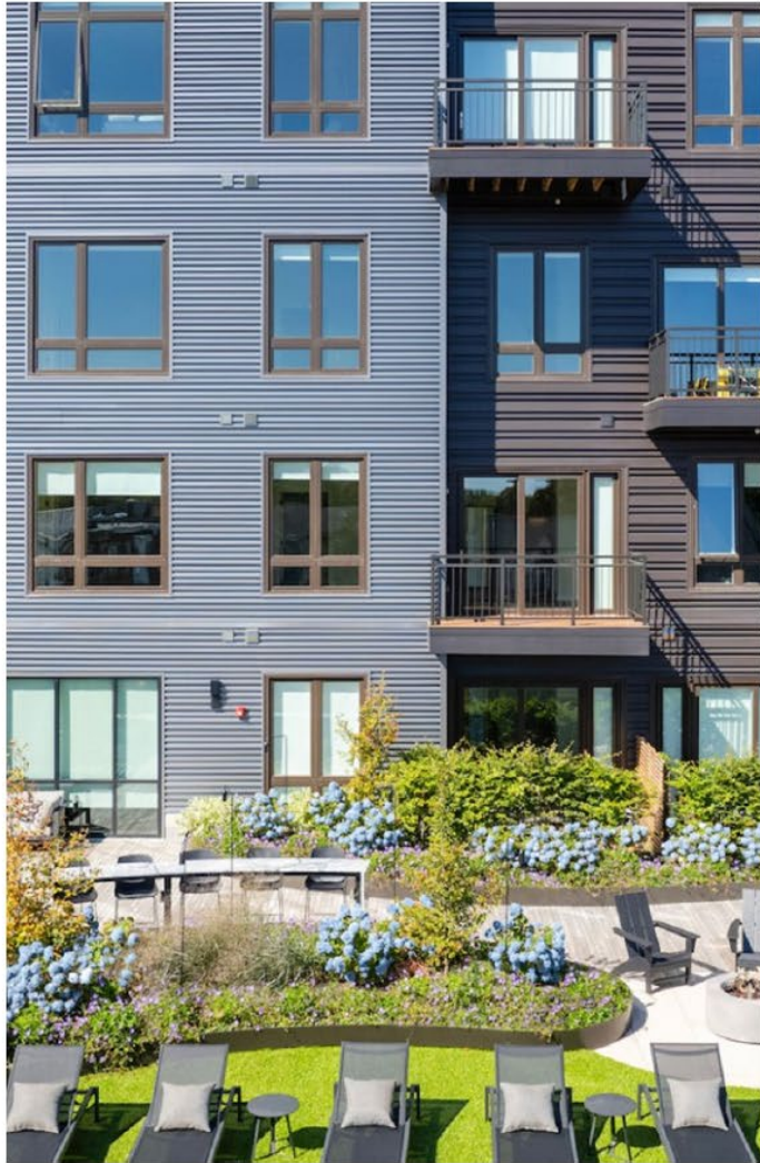
FIBER CEMENT siding at less prominent facades, with varied module sizes to create richness and variety
