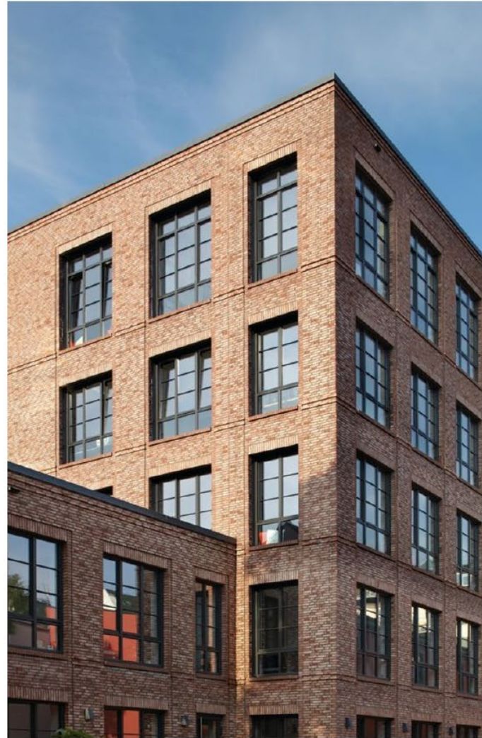
BRICK façade at major elevations of the “Wharf” building, with detailing and simple coursing articulations to pay homage to traditional warehouse buildings in the city.
